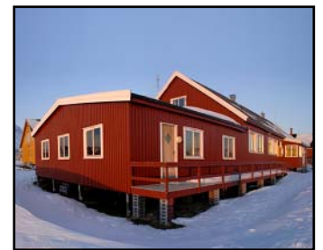
▲ The station at Ny-Ålesund
