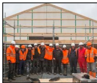
▲ The new building takes shape
